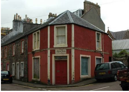
Former Miss Fitz shop premises, possible location of THI office.
